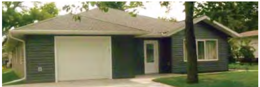
Supported living home at 73 Westwood Drive in Altona
